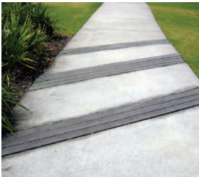
Concrete with timber inserts featuring in entry / nodal areas
